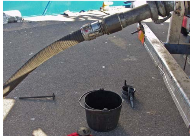
Picture 6: Connection hose to sludgetruck
